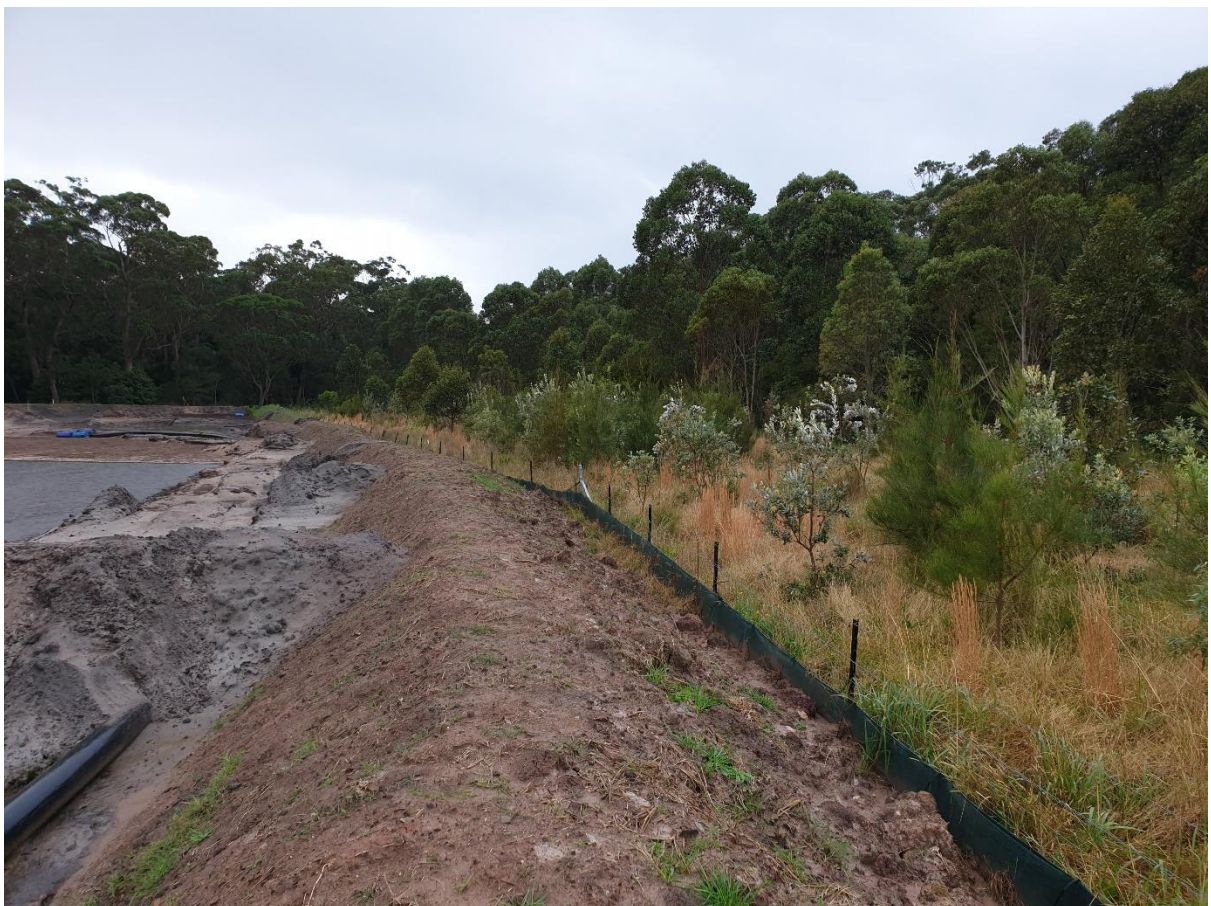
Figure 5 - Flood levee and new dredge pond at northern limit of “CP” area. Revegetation in Zone 2C.1 can be seen in the right side of the photo.
