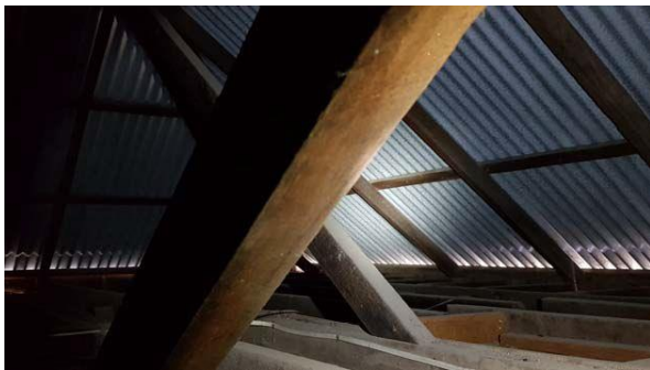
Figure 6: Large Timber Beams in the roof (Source: Design 5, Dilapidation Survey 2018)
