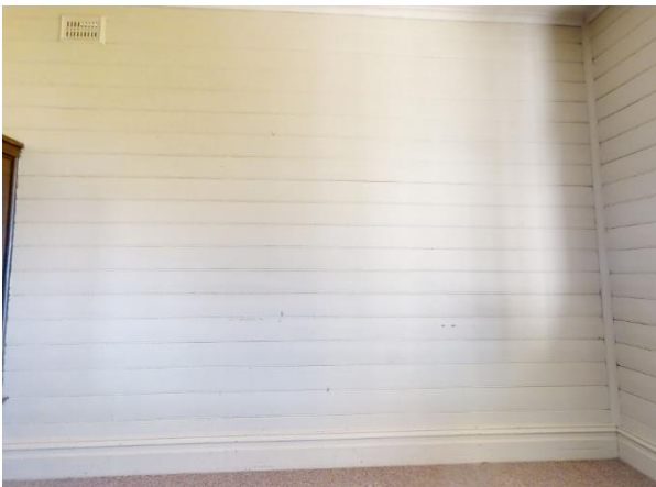
Figure 10: Timber skirting boards (Source: Cleary Bros. 3D Model – The ‘Belmont’)
