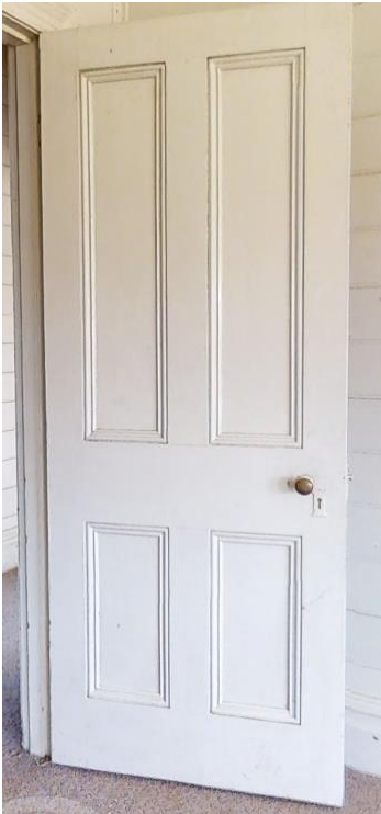
Figure 8: Timber 4-panelled internal doors (Source: Cleary Bros. 3D Model – The ‘Belmont’)
