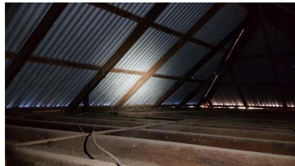
Figure 7: Large Timber Beams in the roof (Source: Design 5, Dilapidation Survey 2018)
