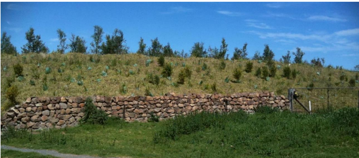
Figure 16: Dry Stone walls, relocated to ‘Belmont’ property entrance, outside of development area in 2010 (Source: HMP 2017)
