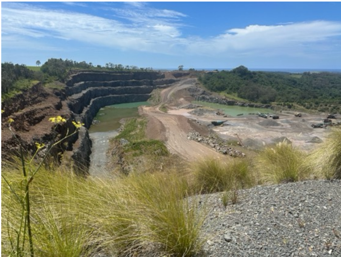
Quarry Active work area showing water sumps.
