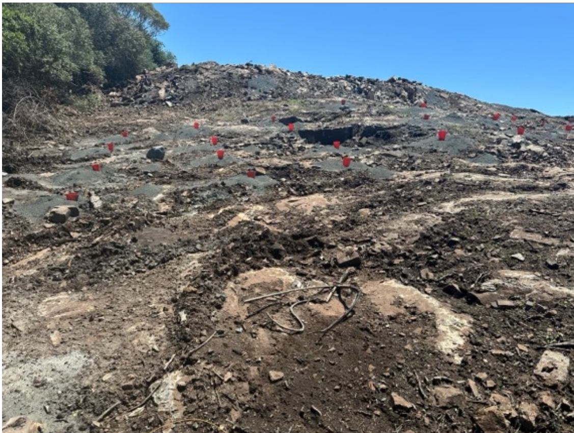
Work area prepared for blasting – Stage 7a
