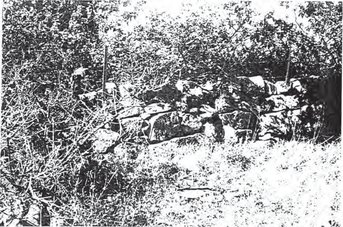
Section C, still intact in most places.
