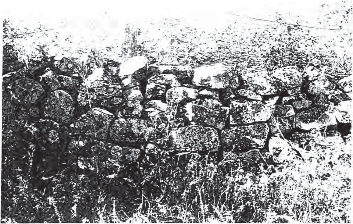
Although still intact this section of wall at Section C shows areas of weakness including running joints
