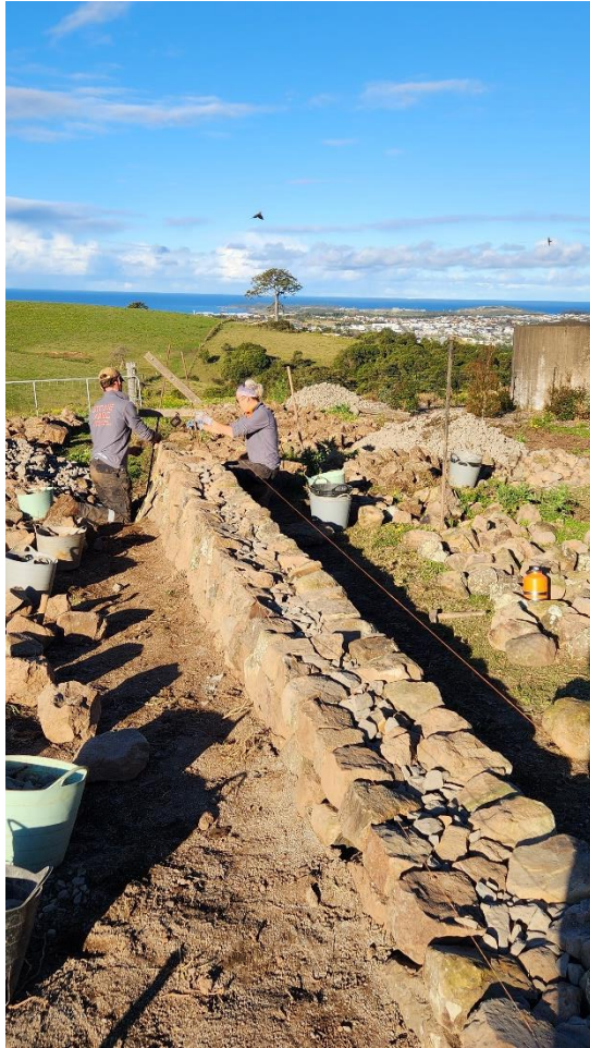
Dry Stone Wall reconstruction underway – August 2025
