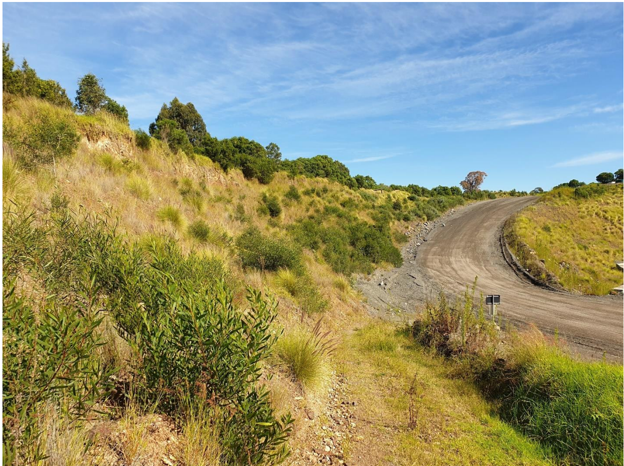
Figure 5 - Southern batter rehabilitation showing establishment of seeded acacia and eucalypts
