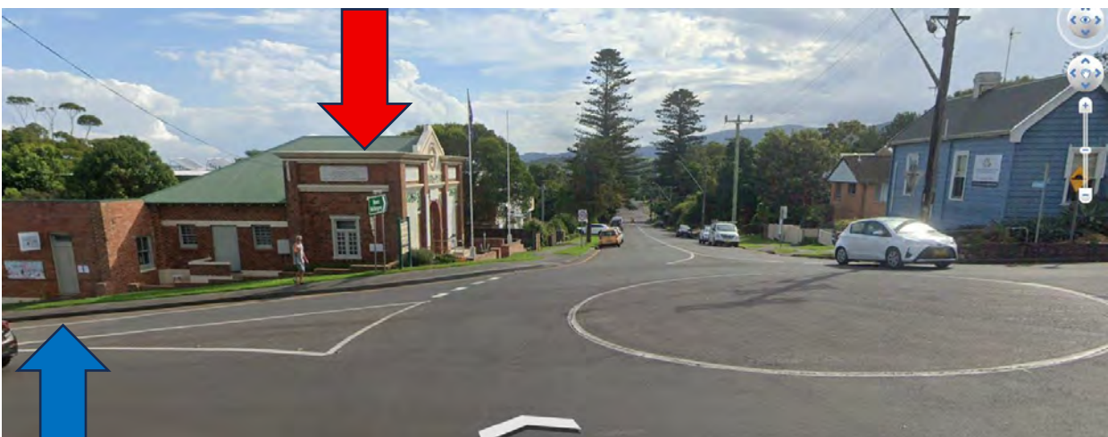
Google Earth – roundabout Fern & Belinda Streets – facing west in Belinda St Fern Street – blue arrow
