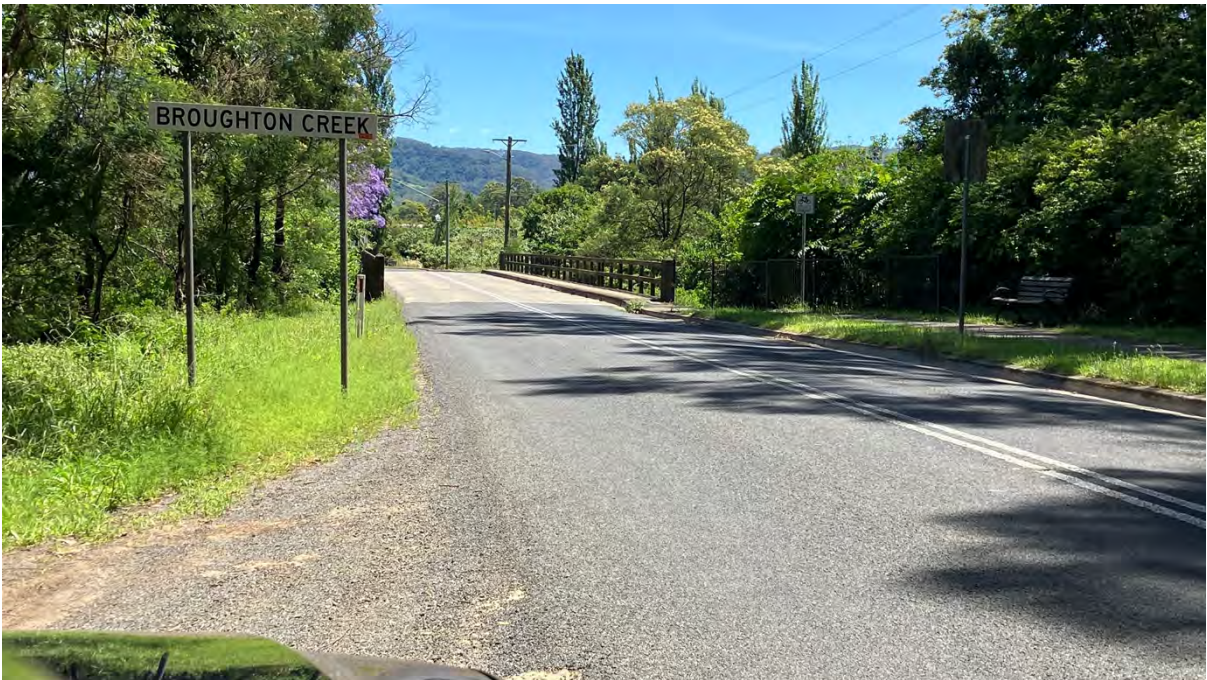
Broughton Creek - Narrow Bridge
