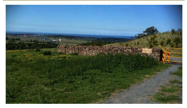
*Figure 7 – Reconstructed dry stone wall adjacent to the Belmont entrance in 2010.*
