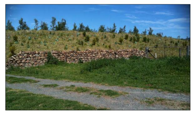
*Figure 6 – Reconstructed dry stone wall adjacent to the Belmont entrance in 2010.*
