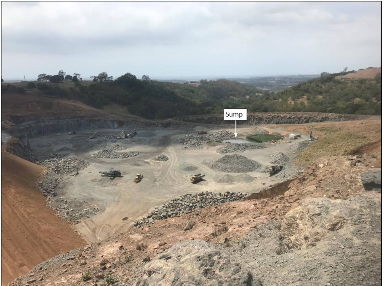
Figure 3.15a: View looking north east, showing extraction area with dry floor/walls, and sump (16/12/2019)
