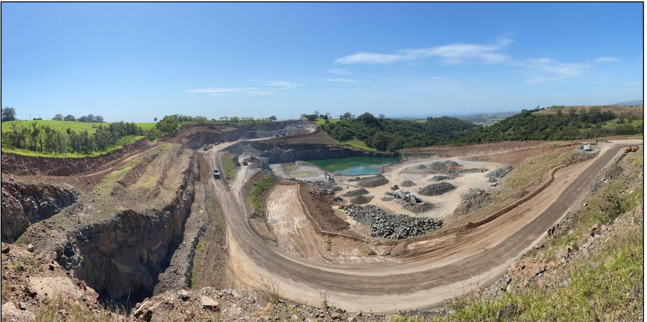
Figure 3.15b: View looking north east, showing extraction area with relatively larger sump that has transitioned to east (16/12/2019)
