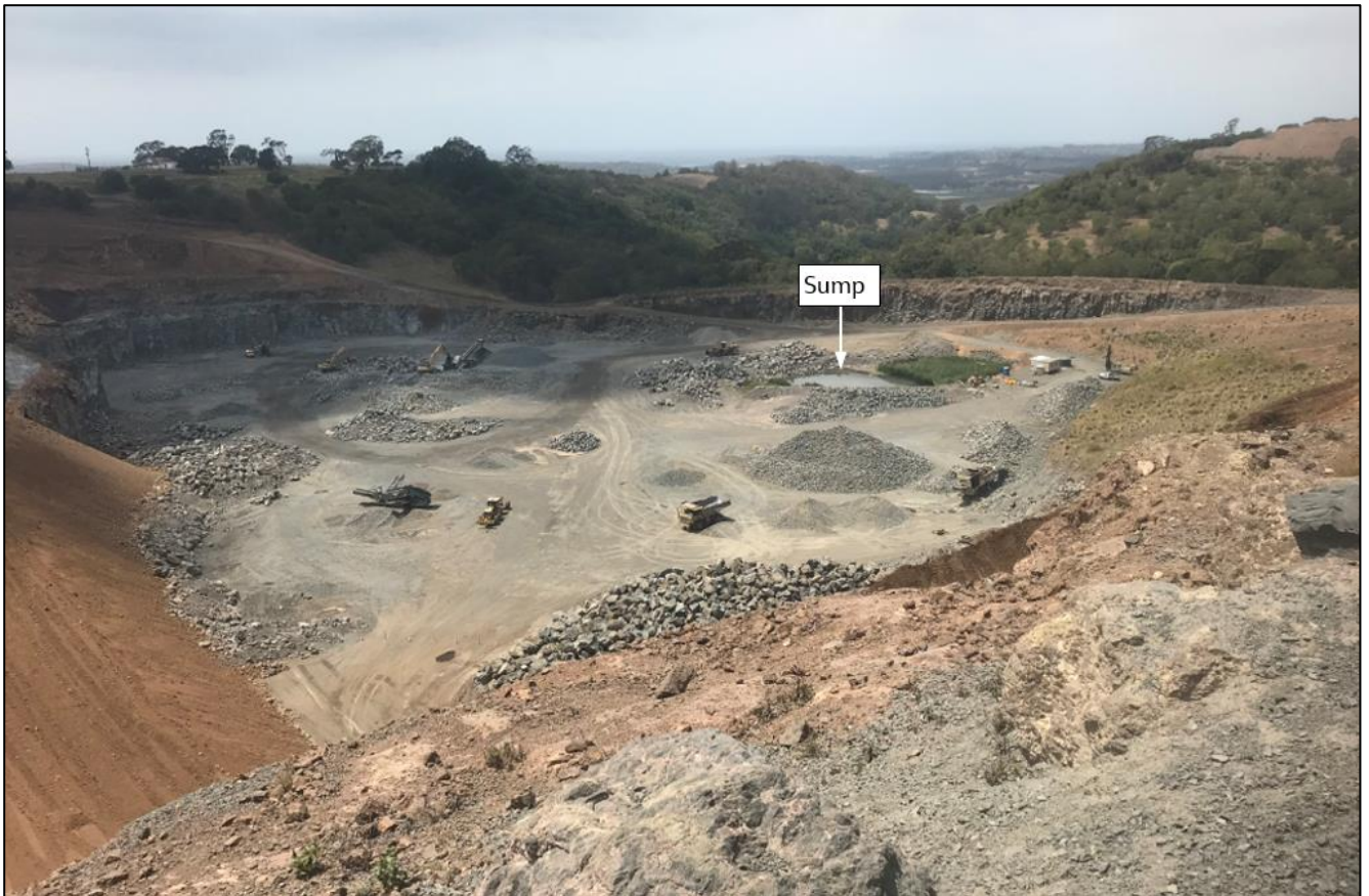
Figure 3.13a: View looking north east, showing extraction area with dry floor/walls, and sump (16/12/2019)
