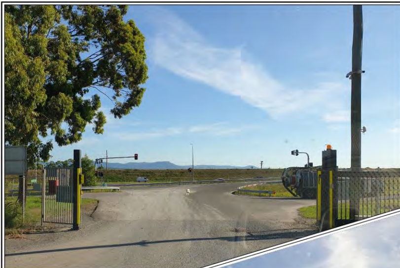
Plate 6.12.1: View of the Site Access Road Looking North forward the East West Link (Source: Cleary Bros)
