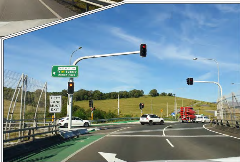
Plate 6.12.6: View of the Oak Flats Interchange, including Signalised Intersections (Source: Cleary Bros)
