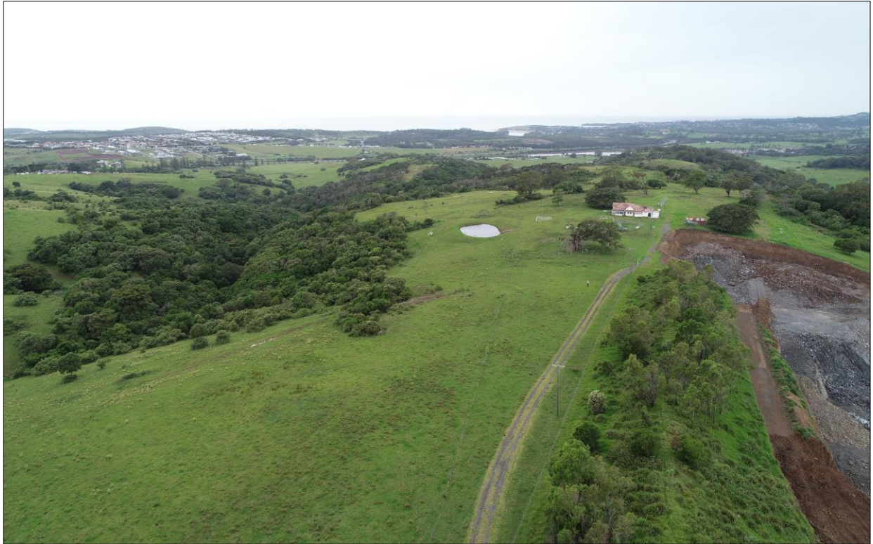
Plate 3.1 Oblique aerial view to the south-southeast across Stage 7 and the current extraction area (Ref: CB-2.7)
