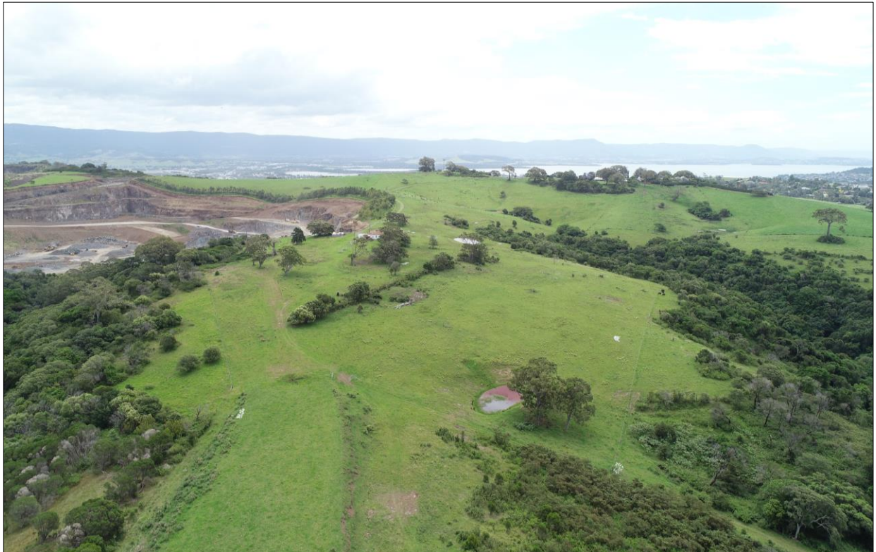
Plate 3.2 Oblique aerial view to the north-northwest across Stage 7 and the current extraction area (Ref: CB-2.9)
