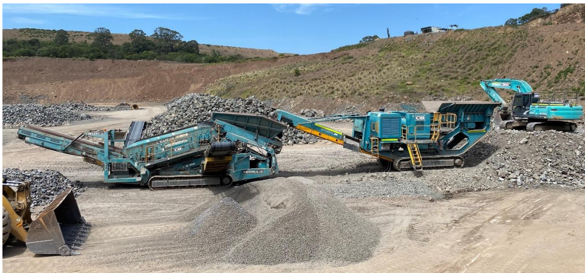
Plate 3.7 Jaw Crusher and Warrior Screen Mobile Plant (Ref: CB-2.10)
