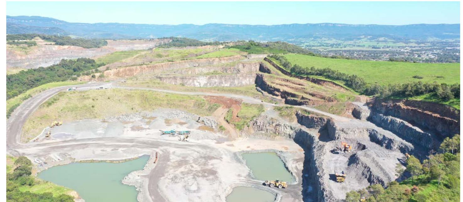
Image 09 - (Drone Image) Views over Albion Park Quarry from the Project Area. (MLA - 02/2023)
