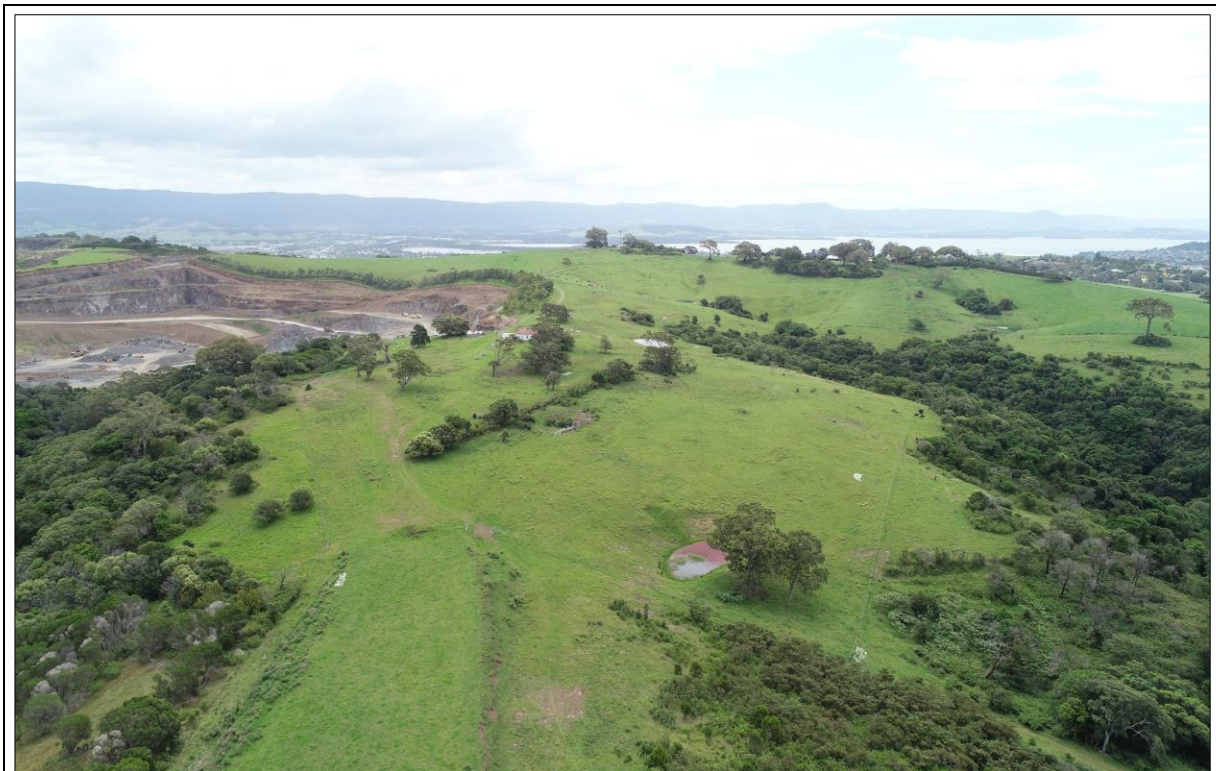
Plate 3.2 Oblique aerial view to the north-northwest across Stage 7 and the current Extraction Area (Ref: CB-2.9)
