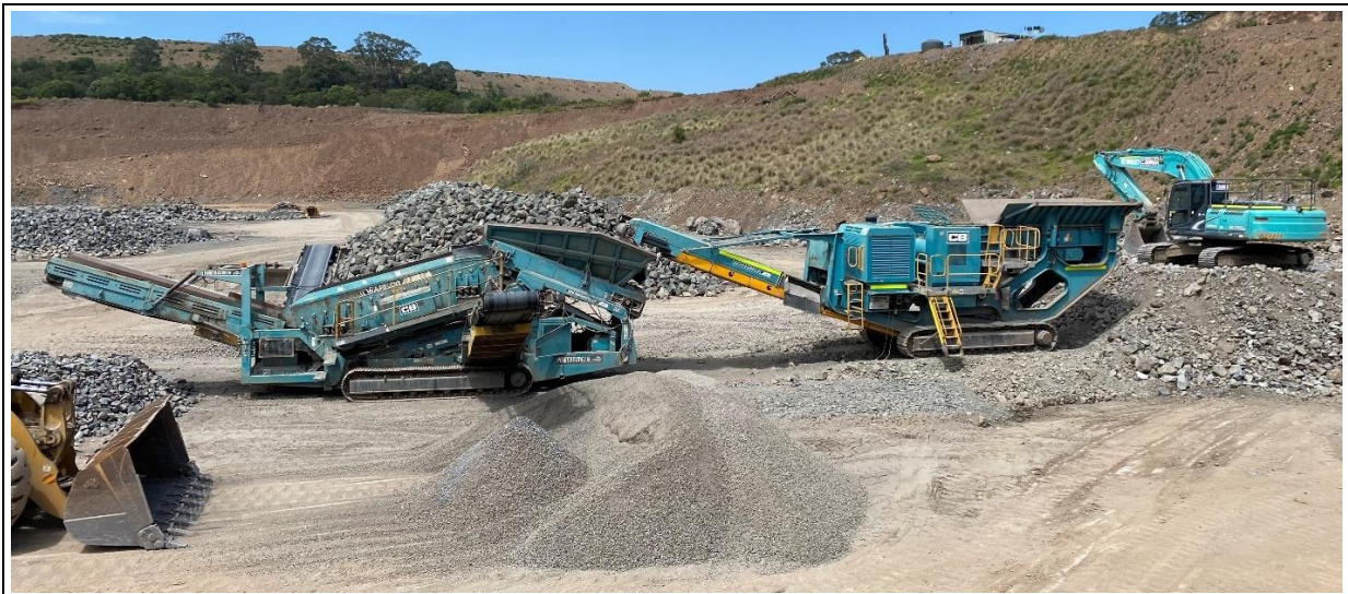
Plate 3.7 Jaw Crusher and Warrior Screen Mobile Plant (Ref: CB-2.10)
